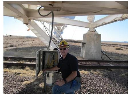
*Mues prepares to disconnect the fiber umbilical from a radio telescope before the antenna is moved to another position in the Very Large Array located near*
